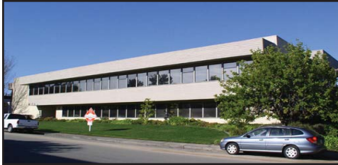
9 Commercial Boulevard Novato
